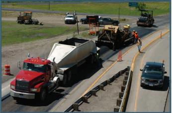
The paver spreads the asphalt, a series of compacting rollers follows.
