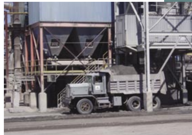
Joliette's landfill practices greatly reduce the size of the waste site and the potential for dust.
